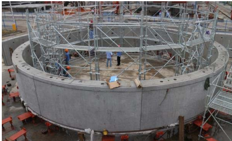
Trail master ring assembly in Dragages Bouygues JV's precast yard (OD13.5m x 2.2m x 0.55m).
